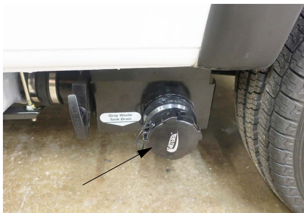
Sewage Drain Outlet (Located beneath motorhome on driver side) - Typical view
